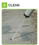
clean the hole thoroughly using a hole cleaning pump and wire brush
