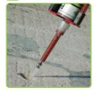
fill the hole 2/3 full with 2202V075 injection resin
